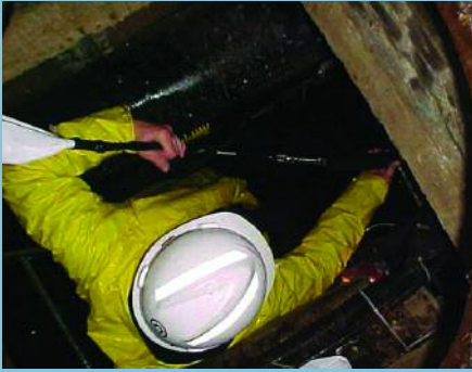
Figure 1: When space is available, this textile innerduct can be placed into any conduit structure.
